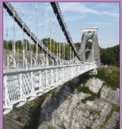
Clifton Suspension bridge
